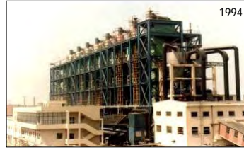
1000 ton per day U-GAS® Industrial fuel gas in Shanghai, China using coal
