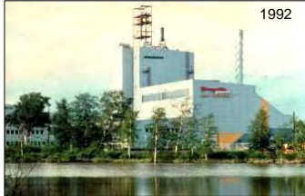
80 ton per day Gasification Pilot Plant in Finland using biomass & coal
