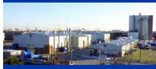
Energy & Environmental Technology Center
