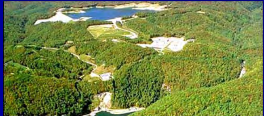
Bad Creek (1065 MW)
