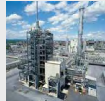
Commercial Gasification Plant
