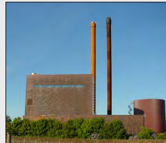
165 ton per day CHP Plant in Skive, Denmark using wood
