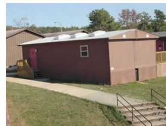
Chapel Hill Middle School (Performance Enhanced Relocatable Classroom)
