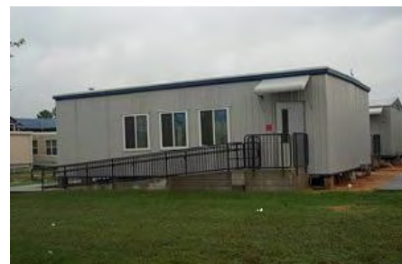
Shingle Creek Elementary School (Performance Enhanced Relocatable Classroom )
