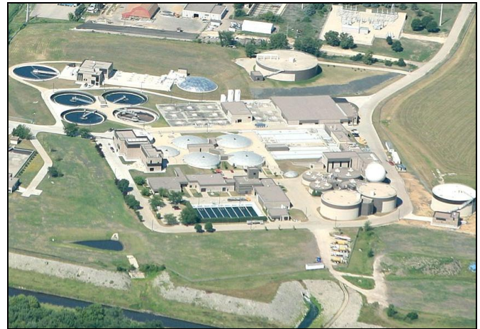
Figure 1: City of Rochester Water Reclamation Plant
