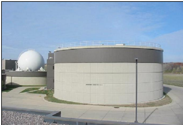
Figure 2: Anaerobic Digester and Gas Sphere
